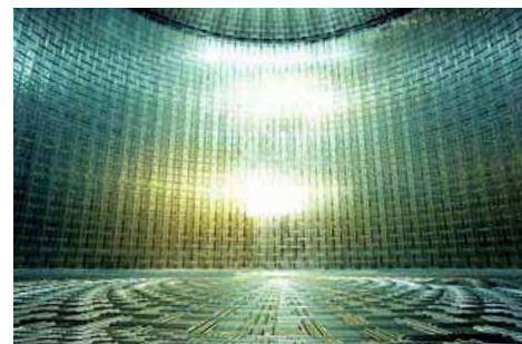
Tokyo Gas's LNG membrane tank in Ohgishima (completed in 1998)
