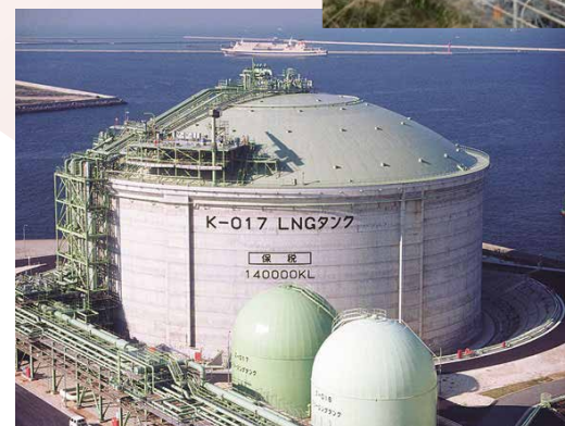
Osaka Gas's PC outer wall LNG tank in Senboku (completed in 1996)
