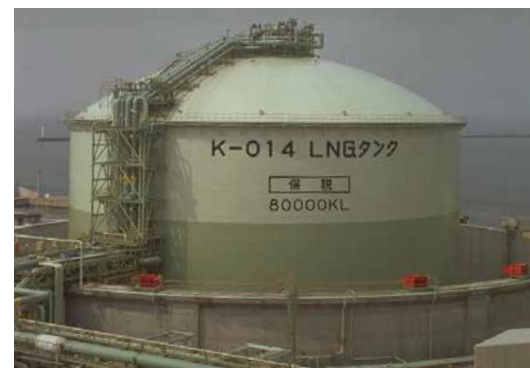
Osaka Gas's double metal wall type LNG tank in Himeji (completed in 1986)
