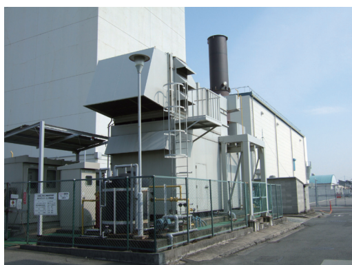
図9 明石工場内発電設備 Fig. 9 Electric power plant at Akashi Works
