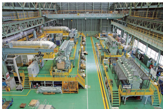
図7 工場試験設備 Fig.7 Factory test facility
