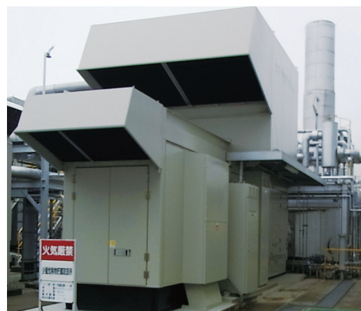
図12 M7A-03搭載発電装置 (PUC80D) Fig.12 Power generation plant (PUC80D) with M7A-03
