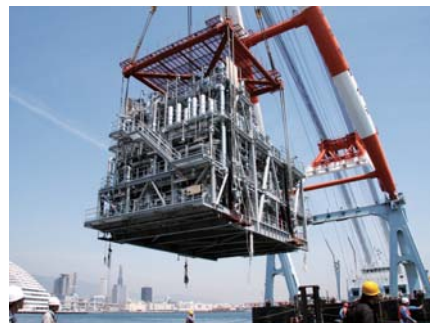
Offshore gas compression module shipped to Korea National Oil Corporation (KNOC)
