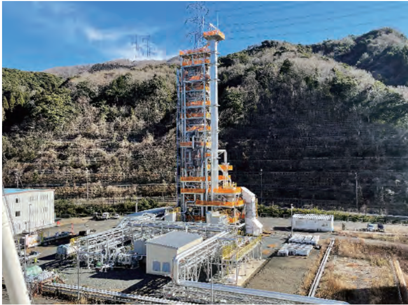
Fig. 5 Pilot-scale moving bed solid sorbent plant
