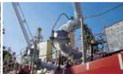
The loading arm is completely frosted over due to the cryogenic temperature.
