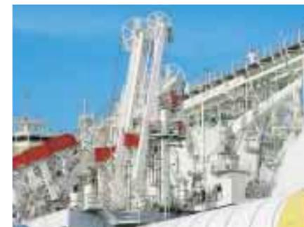
Unloading arm. LNG is discharged through these pipes.
