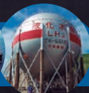
Long term storage of liquefied hydrogen
