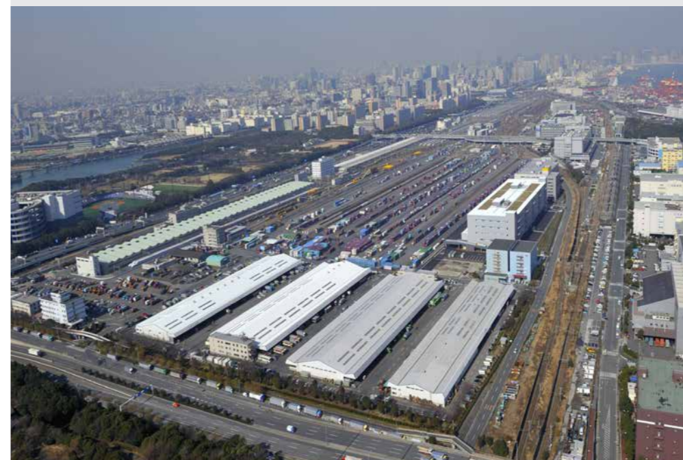
Tokyo Freight Terminal Station serves as one of JR Freight's transport hubs (located in Shinagawa Ward, Tokyo)
