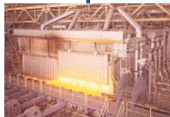
炼铁用液压装置 Hydraulic equipment for steel making plant
