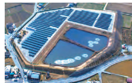
Kawasaki Trading Co., Ltd. Iwaoka Photovoltaic Power Generation Station: 1,505-kW power generation facility
