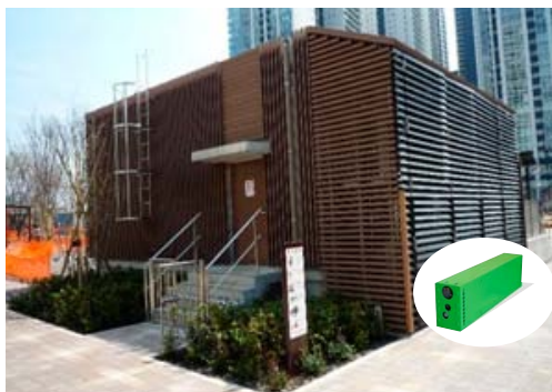
Railway battery power system
