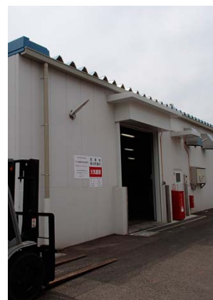
PCB storage warehouse
