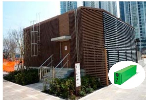
Railway battery power system
