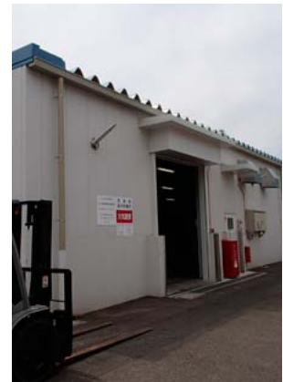
PCB storage warehouse
