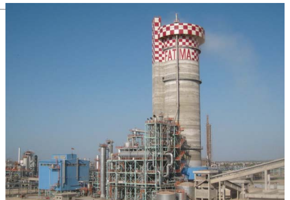
Urea manufacturing facility
