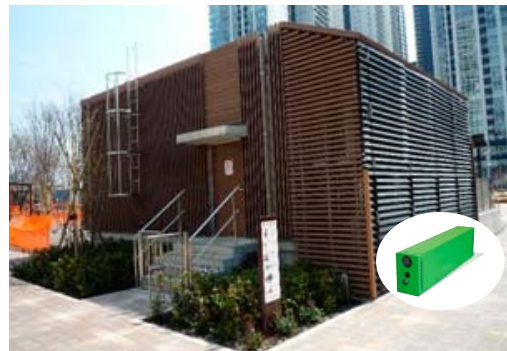
Railway battery power system
