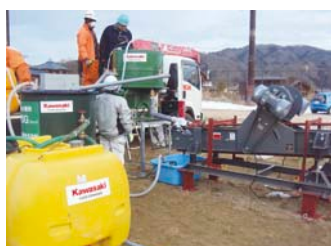
Soil remediation verification test
