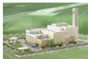
Waste Incineration Plant
