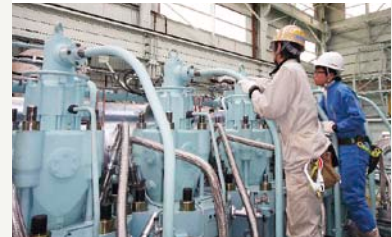
Shop test of critical equipment
