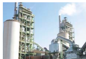
Cement plant waste heat recovery power generation
