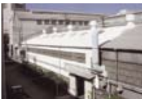
Plant Building with Heat Insulating Paint
