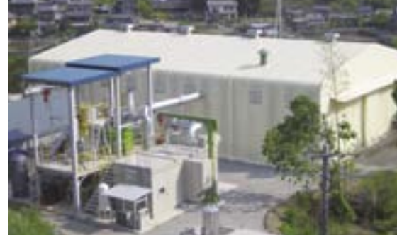
Test plant in Niyodogawa, Kochi Prefecture
