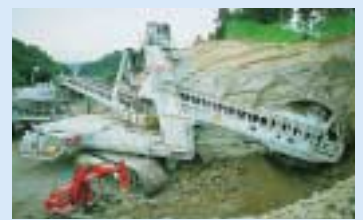
Bucket wheel excavator (BWE)
