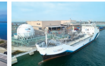
Liquefied hydrogen cargo handling demonstration terminal and liquefied hydrogen carrier, SUIISO FRONTIER
