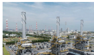
KG-18-T 100 MW-class combined cycle power plant
