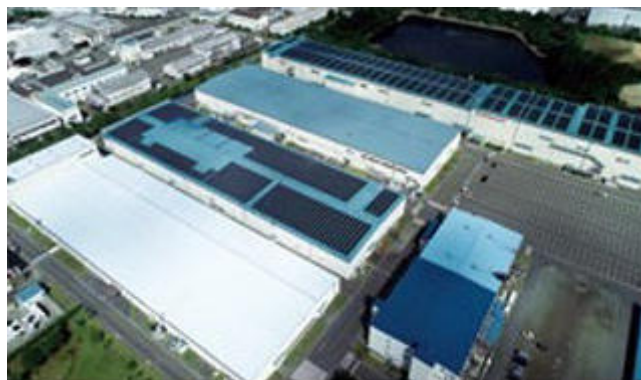
Seishin Works: 728-kW power generation facility
