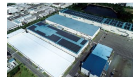
Figure 15: Seishin Works: 728-kW power generation facility
