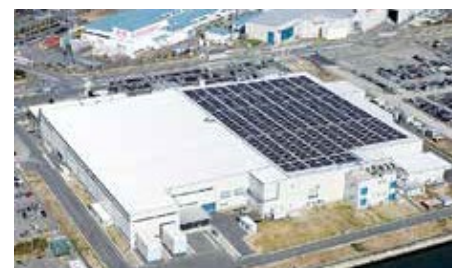
Figure 14: Nagoya Works 1: 750-kW power generation facility
