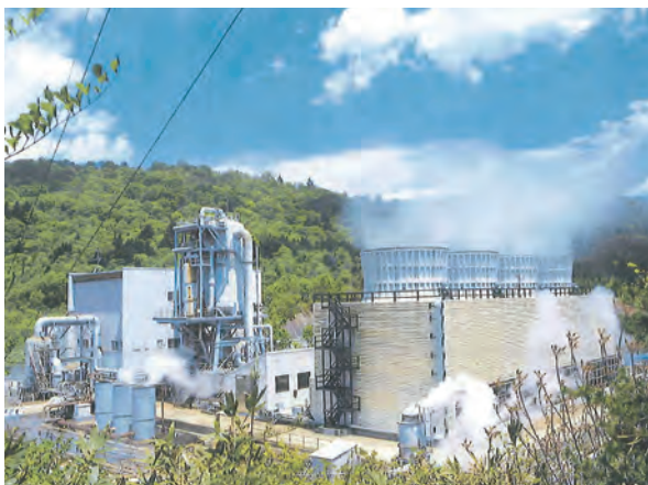
Fig. 3 Geothermal power generation facility
