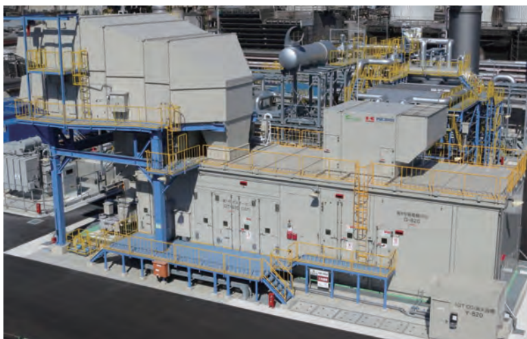
Fig. 3 30 MW class PUC300 cogeneration facility
