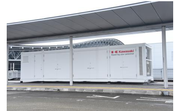
Container installed at Kansai International Airport
