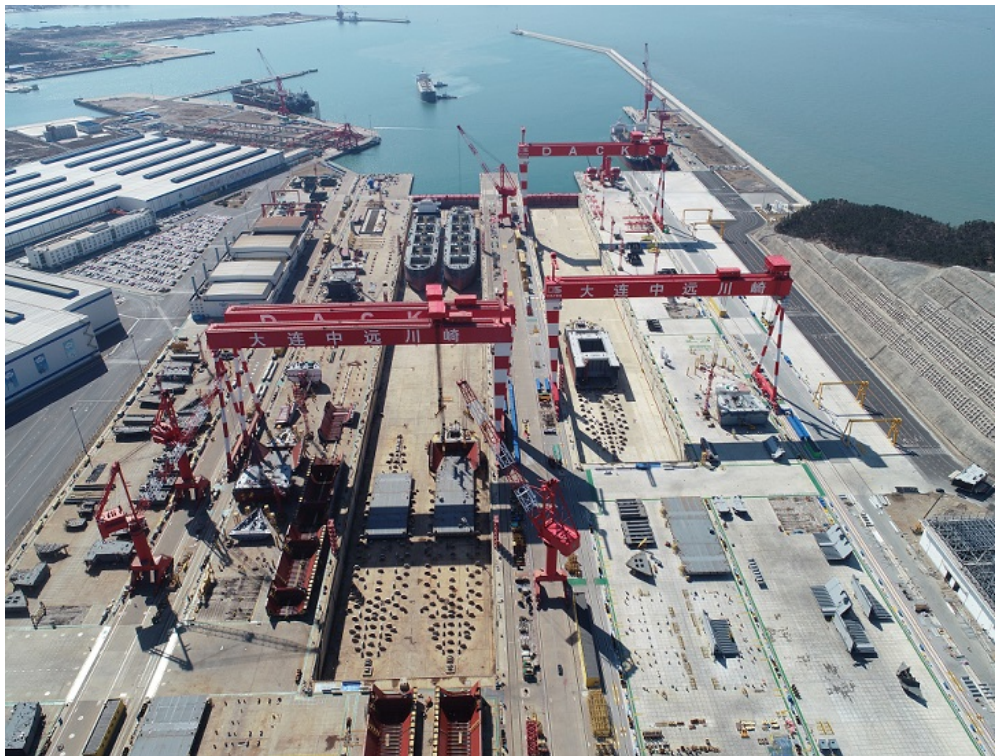
DACKS factory panoramic view. Right dock is the second dock.
