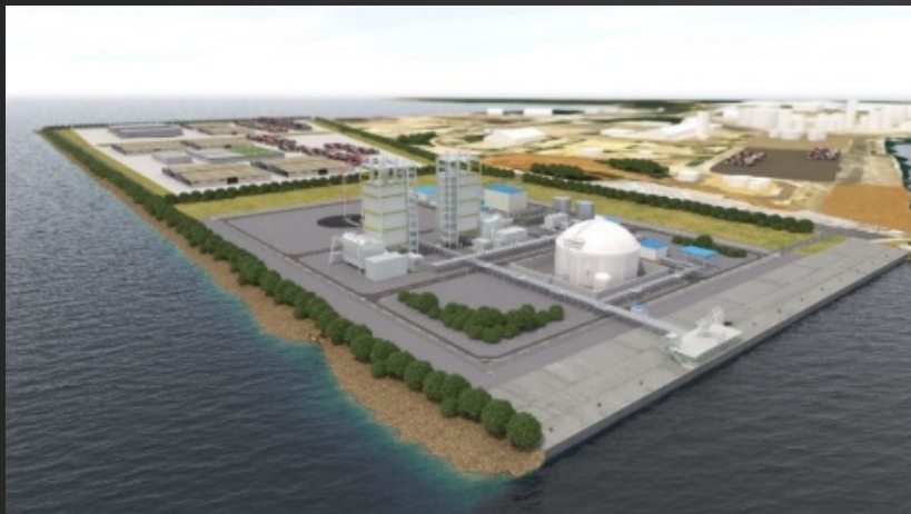
Liquefaction and Loading Terminal (50,000 m 3 x 1 hydrogen tank)
