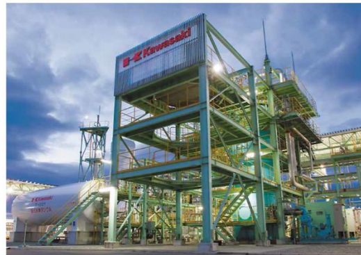
Hydrogen liquefaction plant demonstration facility built at Harima Works
