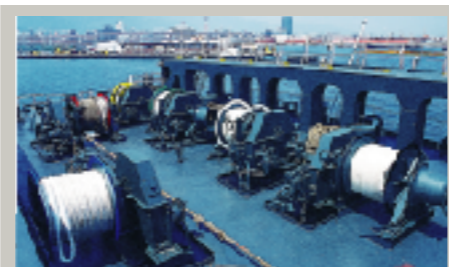
泊船绞盘 Mooring winch
