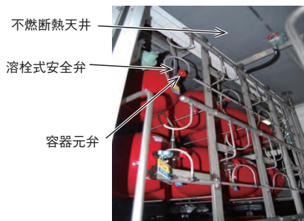
図4 中央部容器元弁操作室 Fig.4 Central vessel master valve control room
