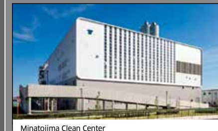
Minatojima Clean Center (operated by Kobe City Environment Bureau)
