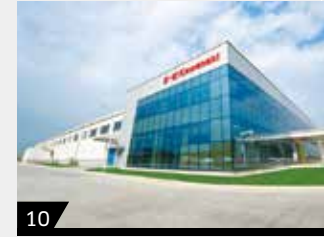
10 Kawasaki Precision Machinery (Suzhou) Ltd. (Suzhou, China) •Area: 91,773 m 2 •Products: Hydraulic pumps, motors, valves, and other hydraulic equipment
