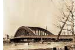
1926 Constructs Eitaibashi Bridge, Tokyo
