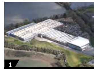
1 Kawasaki Precision Machinery (U.K.) Limited (Plymouth, U.K.) •Area: 68,800 m 2 •Products: Hydraulic pumps and motors, other hydraulic equipment
