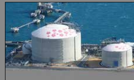
LNG storage tank (left), LPG storage tank (right)
