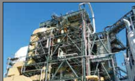
U-KACC boiler and turbine generator
