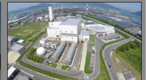
Waste treatment and biogas generation complex
