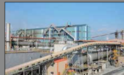
Nonferrous metal (ferronickel) plant
